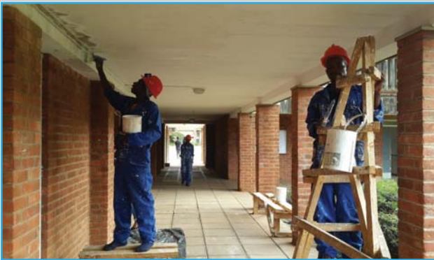
Painters revamping the look of the college corridors
