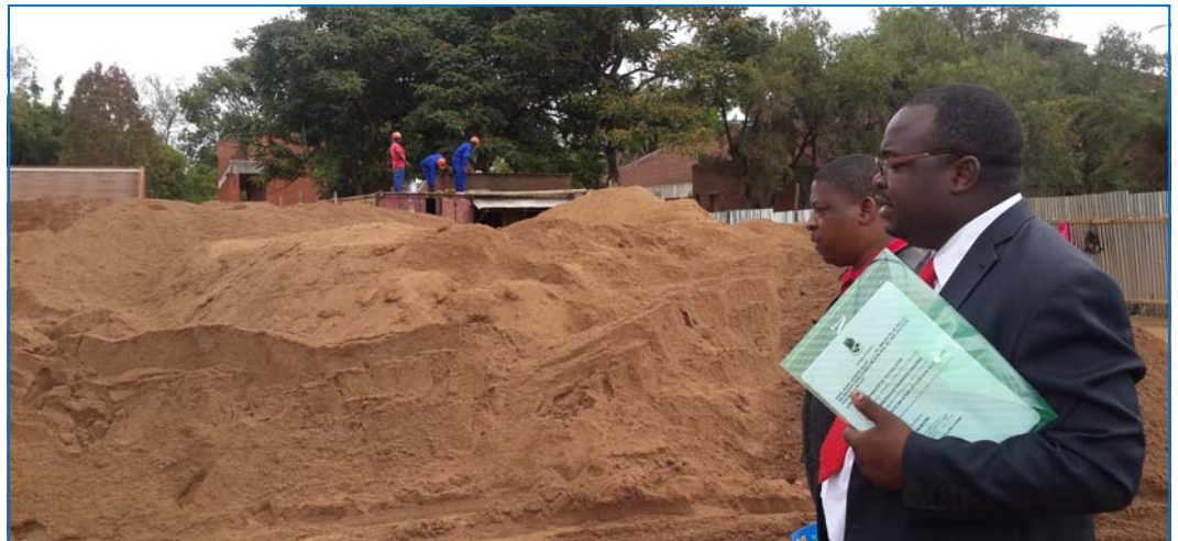
The Principal leads the Reform Team through one of the construction sites
