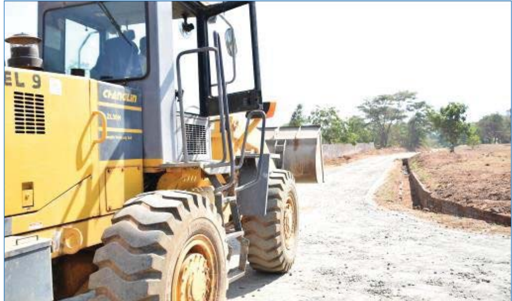
A bulldozer working on the road
