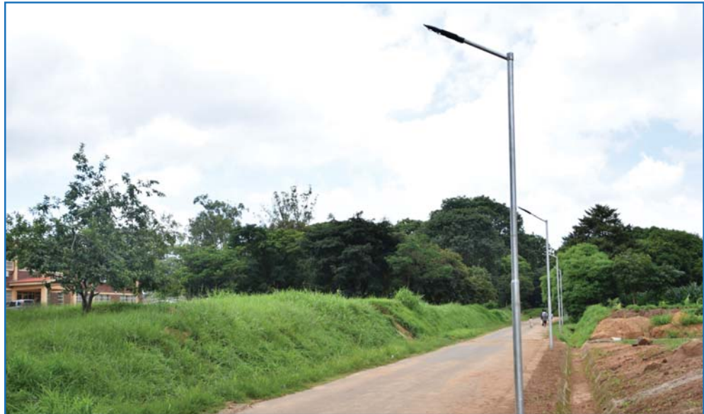
The new street lights
