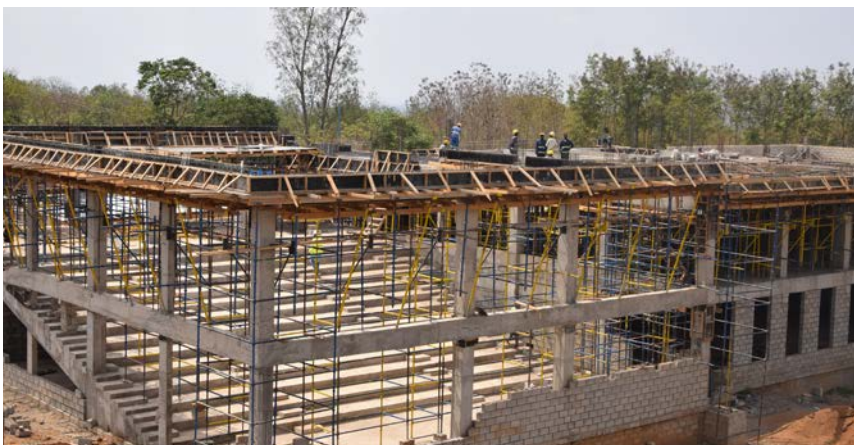
Construction of lecture theatres
