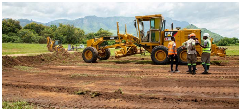
Some of the equipment brought by Zipatso Ltd to the site
