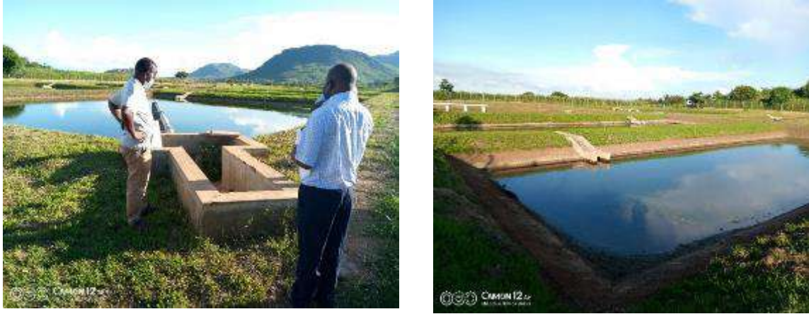
Figure 5.3 Wastewater stabilization ponds at University of Malawi
